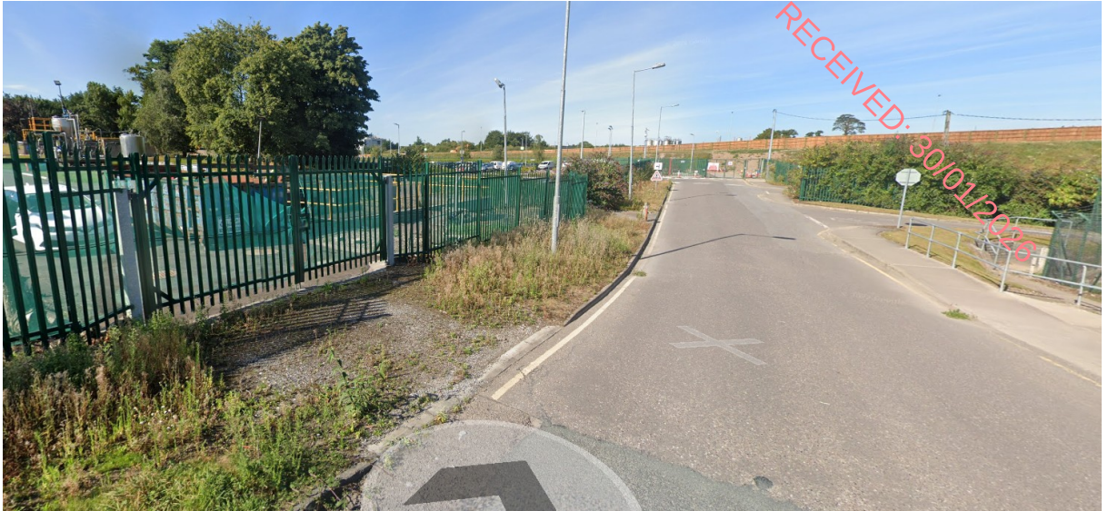
Primary construction plant & delivery access via existing western gate
